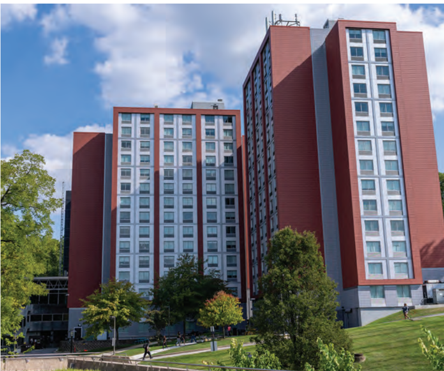
Glen Tower Complex in 2026
